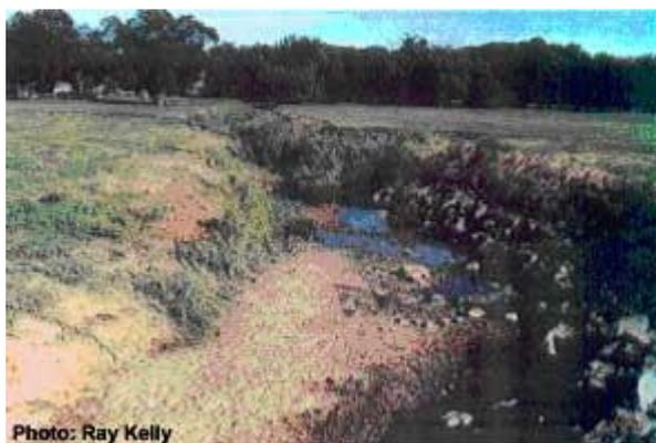
**Fig. 12** July 1997 Erosion control work placed to stabilise the north bank. concrete block used as a position reference was removed during these works
